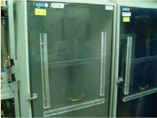
Cubicle For Tests
