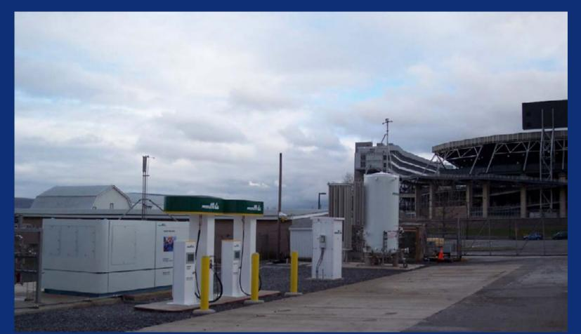
LHy supply system, H2 compression, H2 storage, H2 dispenser and Blend dispenser installed Oct. 2004.
