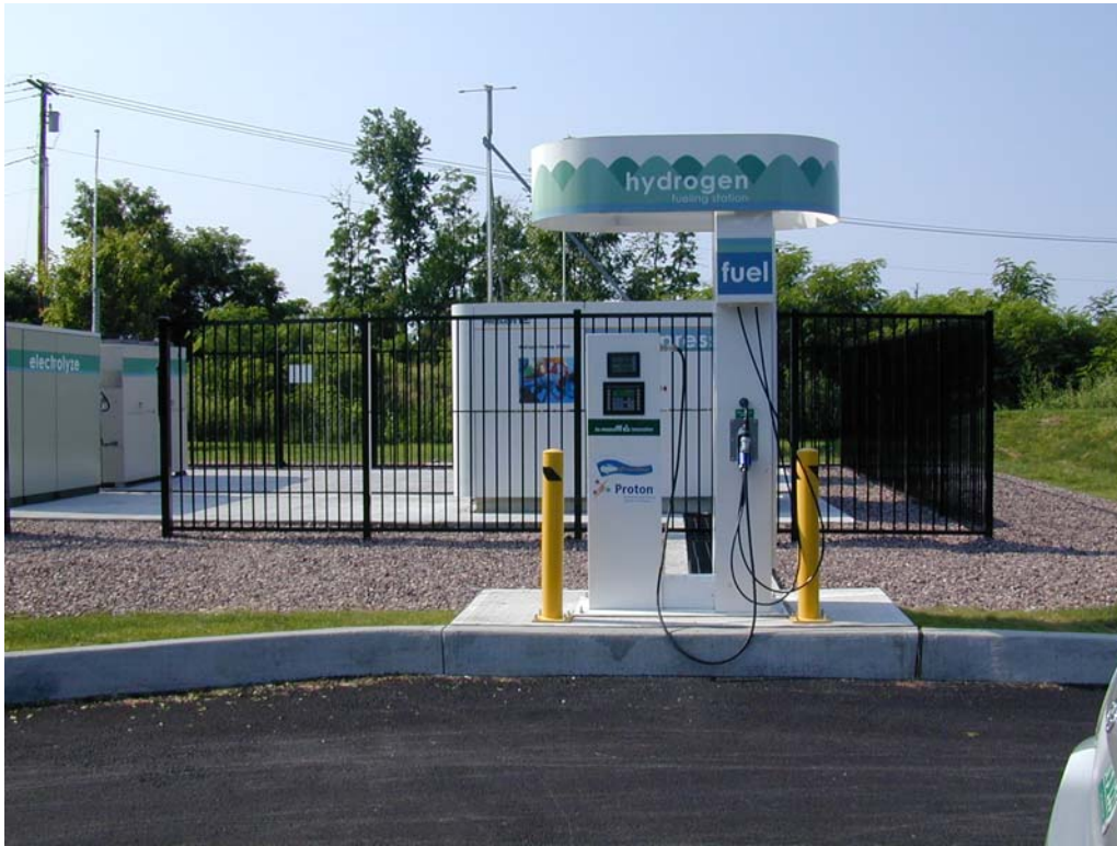
Fueling Station Site June 2006 at Burlington (VT) Department of Public Works
