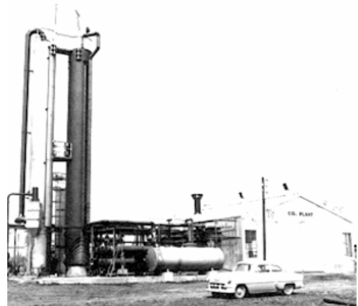
Early GEECO CO 2 Plant
