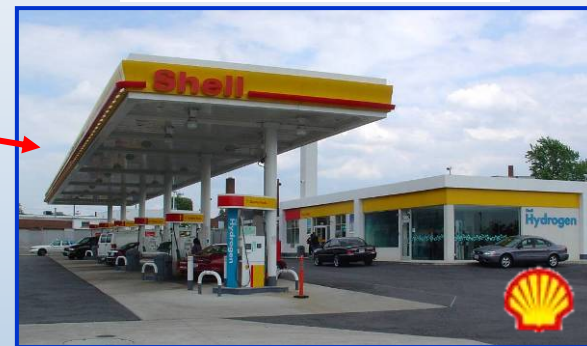
Hydrogen and gasoline station Washington, DC
