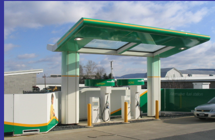
Hydrogen Filling Station
