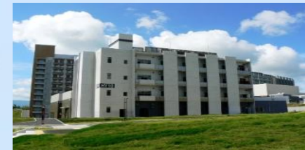
HYDROGENIUS Main building
