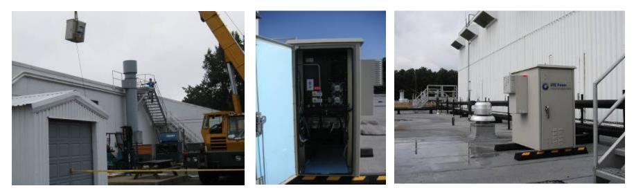
**Application:** supply emergency backup power to security and emergency response radio repeaters.
