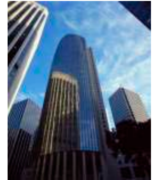
Commercial Power Stationary Power Units
