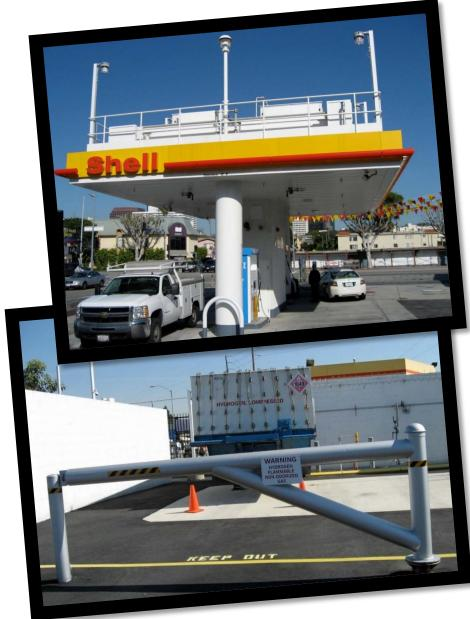
Shell's 350-bar West LA. station is very compact with H2 storage above a shared gasoline/hydrogen island.
