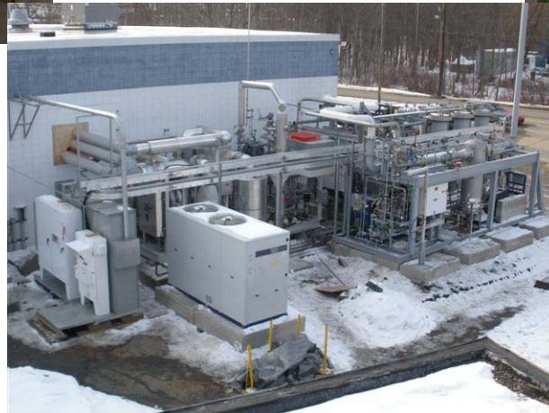
Anode Exhaust Processing and H 2 Purification System
