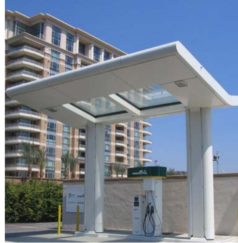
The UC Irvine Fueling Station operated by the National Fuel Cell Research Center (NFCRC) photo by Lorin Humphries.
