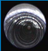
Dynalene FC (no deposits or corrosion debris)
