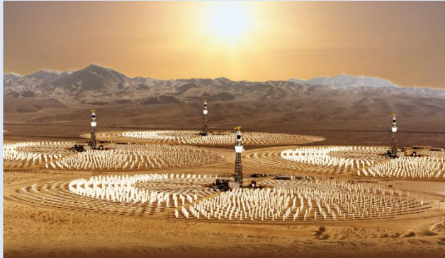
A solar concentrator uses mirrors and a reflective or refractive lens to capture and focus sunlight to produce temperatures up to 2,000°C. This high-temperature heat can be used to drive chemical reactions that produce hydrogen.
