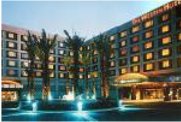
Westin at SFO Airport Nat Gas CHP
