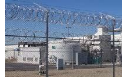
Santa Rita Jail, CA Nat Gas Fuel Cell and Solar Power
