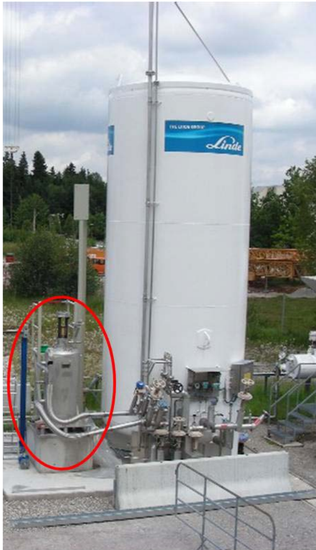
BMW high pressure cryogenic pump
