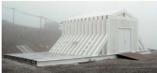
Blast-hardened Sub-Scale Warehouse at SRI Test Site
