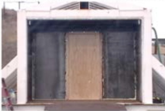
Sub-Scale Warehouse Showing Plywood Pressure Relief
