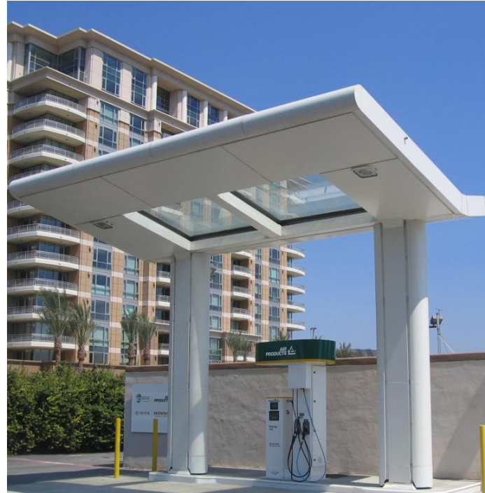
The UC Irvine Fueling Station operated by the National Fuel Cell Research Center (NFCRC) photo by Lorin Humphries.
