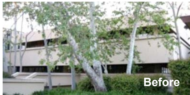
Jorgensen Laboratory Building
