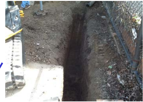
3/11 water/communication trench
