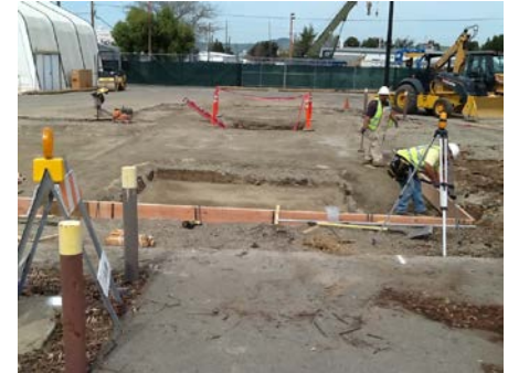
3/20 Equipment pad preparation
