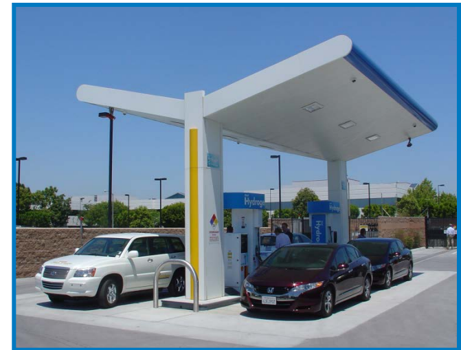
APC/Shell Pipeline station, Torrance, CA. Photo: NREL
