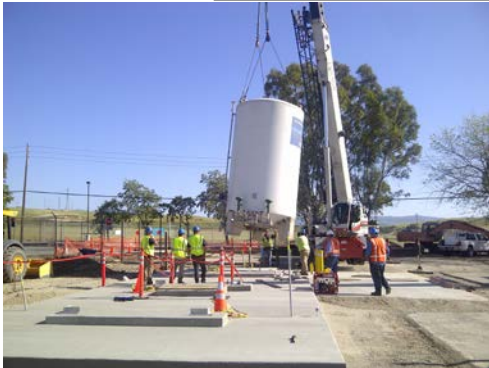
Dewar and pump installation
