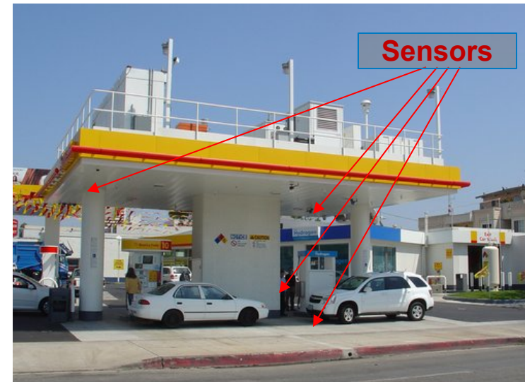
Hydrogen dispenser equipped with wall-mount and internal sensor
