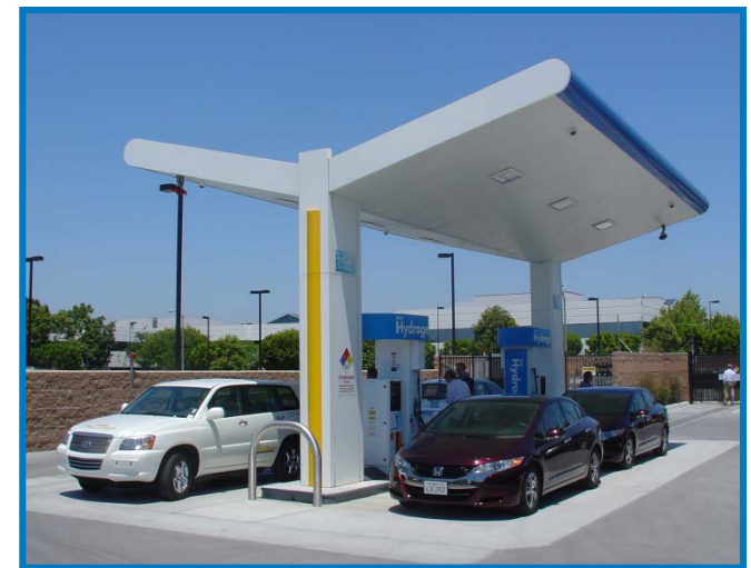
APC/Shell Pipeline station, Torrance, CA. Photo: NREL
