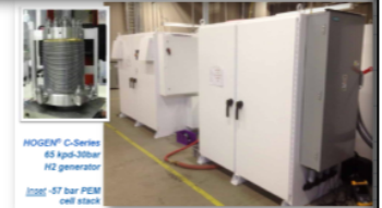
Figure 1. SunHydro #1 Compression, Storage, Dispensing Containerized System
