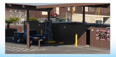
Fill on-site at the end of Pier 39 with a hydrogen delivery service (Luxfer-GTM)
