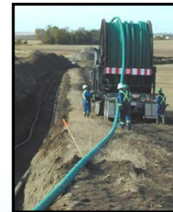
Spooled FRP Installation
