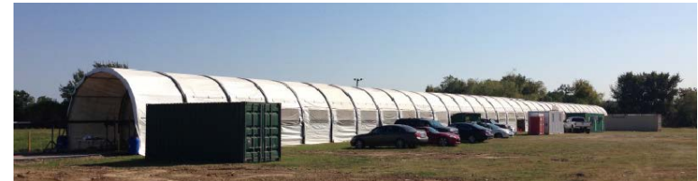
Site Manufactured FRP
