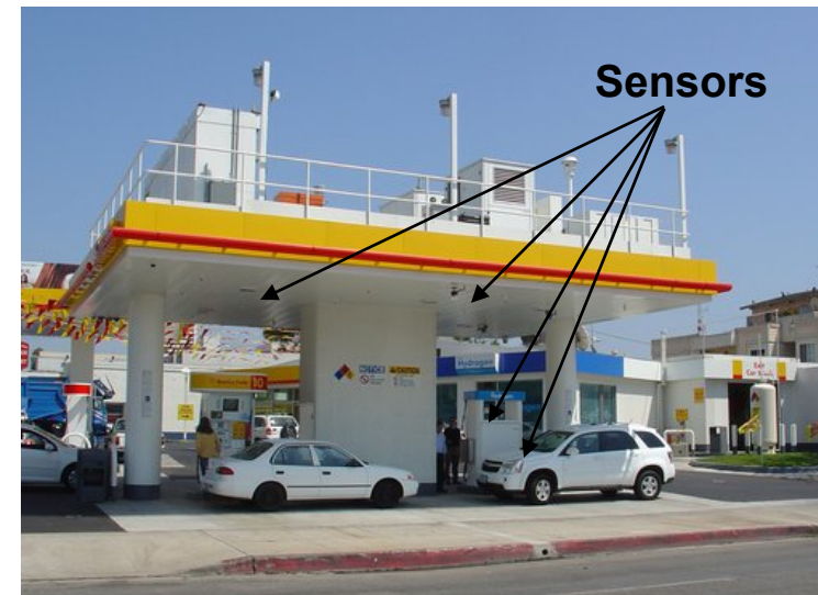
Hydrogen dispenser equipped with wall-mount and internal sensors
