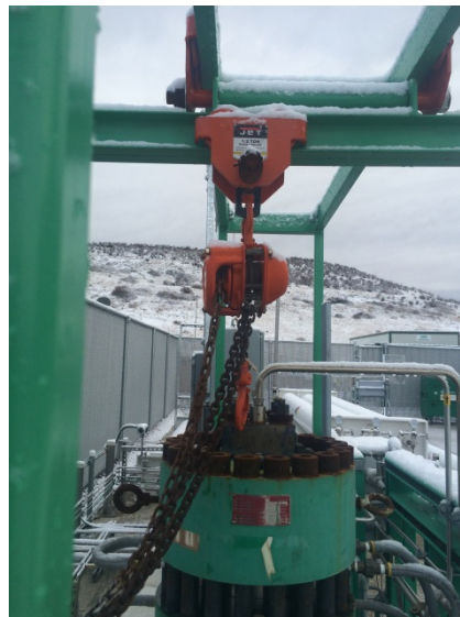
On frame hoist
