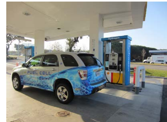
Shell Newport Beach station built by Powertech
