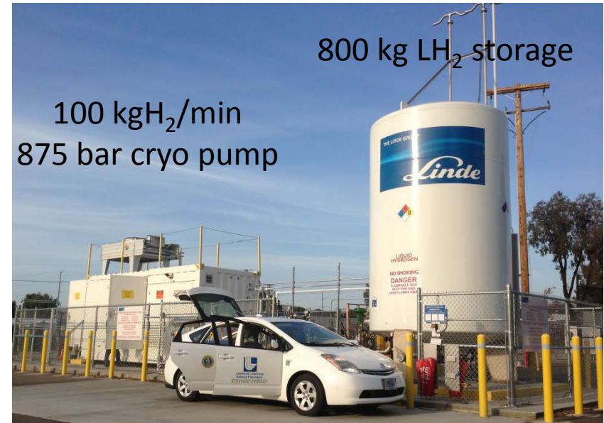
7 minute 10 kgH 2 fill to 70 g/L (350 bar, 65 K)
