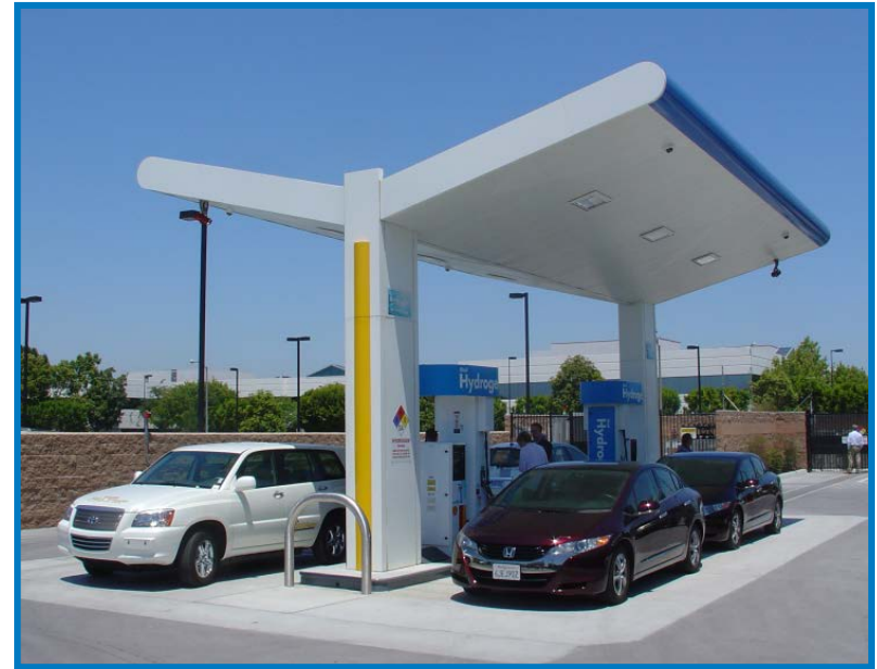
APC/Shell Pipeline station, Torrance, CA. Photo: NREL
