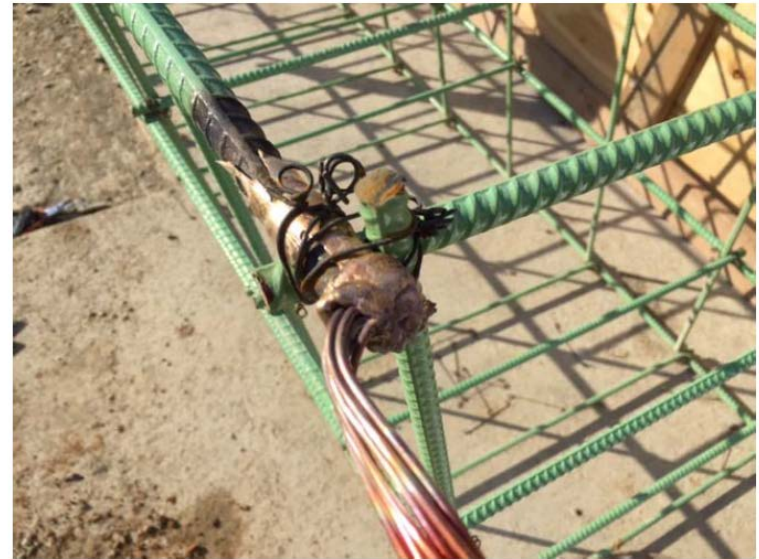
12 Grounding bar attached to steel rod reinforcement.
