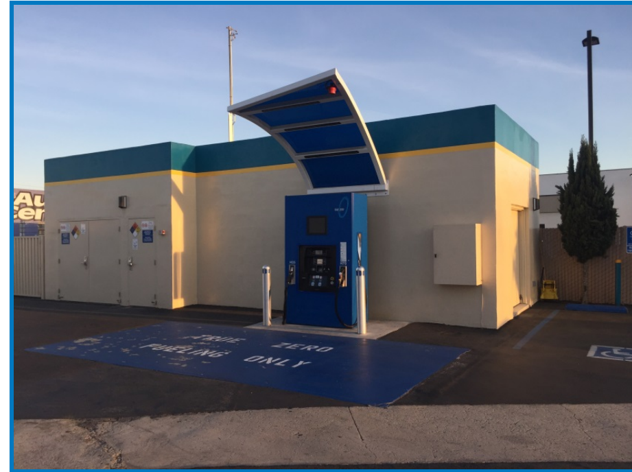
First Element, Costa Mesa, CA. Photo: NREL
