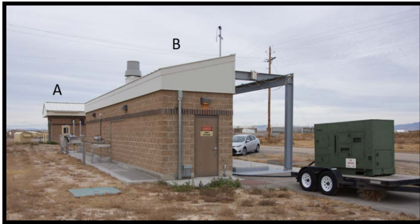
MHAFB headworks buildings—inlet & grate (A), grinder & pumping station (B)
