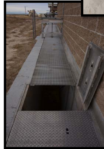
Open channel post grinder, pre-pump station
