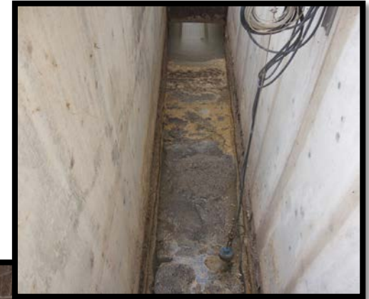
Open channel post grinder, pre-pump station
