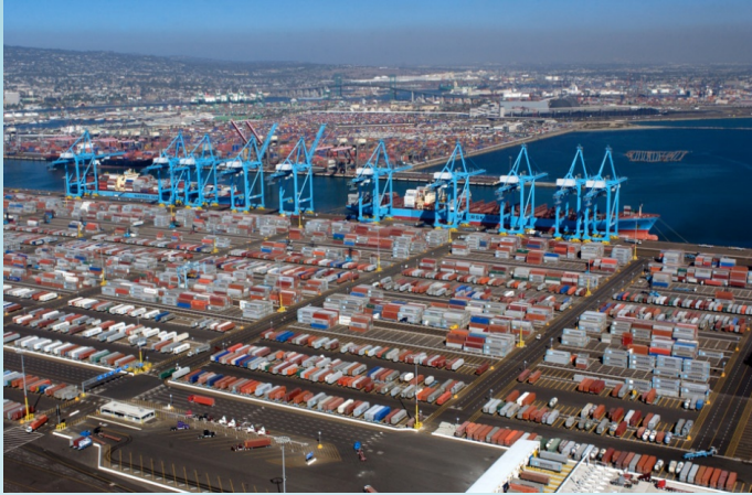
Port of Los Angeles, California
