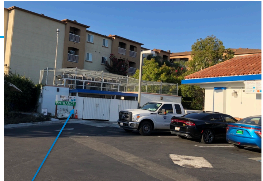
Hydrogen fueling site storage area with space constraints
