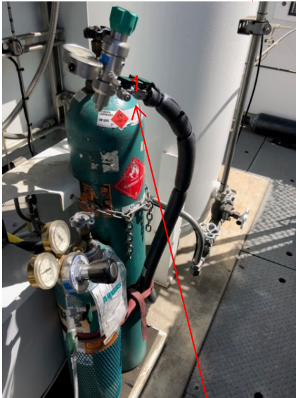
Insulation applied
