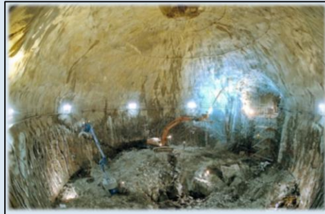
Cavern Excavation + Drainage
