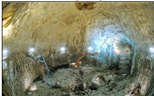
Rock excavation (dome), Skallen,
