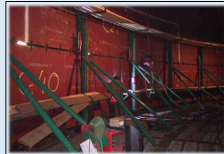
Liner installation
