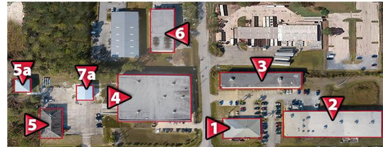
1 - ENGINEERING OFFICES 4 - PRODUCTION FACILITY 6 - ADMINISTRATIVE OFFICES 2 - RESEARCH & DEVELOPMENT 5 - PRODUCT DEVELOPMENT 7a - ROTOMOLD PRODUCTION - 1 3 - RESEARCH & DEVELOPMENT 5a - MAINSTREAM EBEAM
