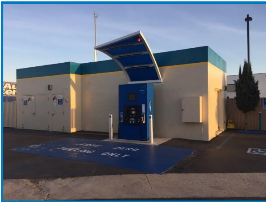
FirstElement Fuel, Costa Mesa, CA. Photo: NREL
