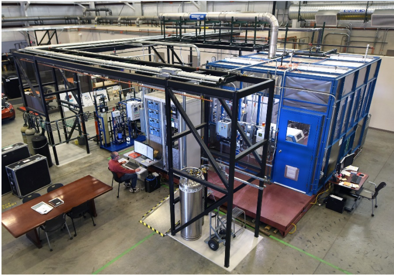
25 kW HTE Test Facility Overview in DETAIL within the INL Energy Systems Laboratory
