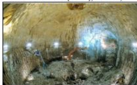
Rock excavation (dome), Skallen,
