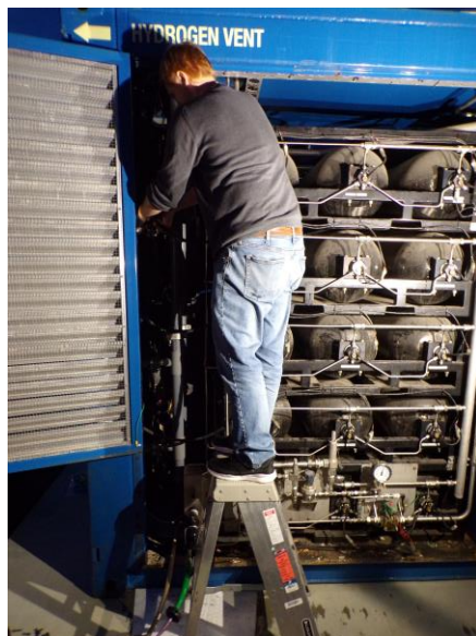
Max Muller (Hydrogenics/Cummins) removes broken PVC piping
