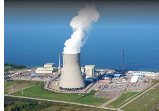
Nine Mile Point Nuclear Power Plant
