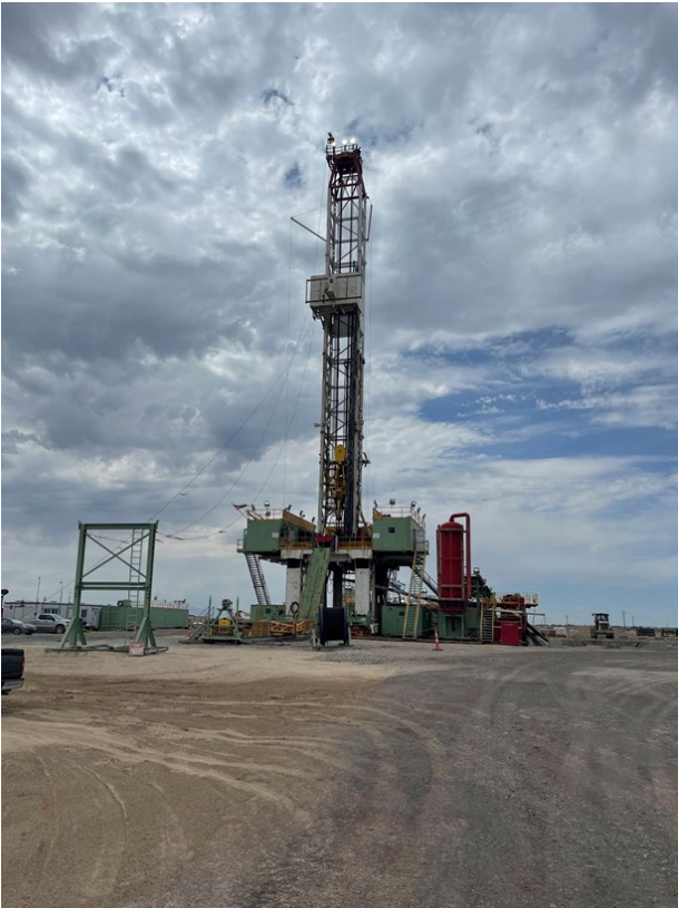
Drilling Rig Mobilized – Drilling started
