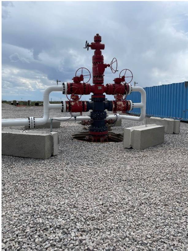
Drilling Complete – Solution Mining Started
