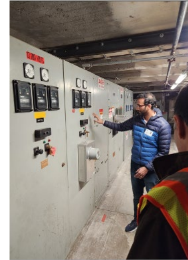
Raman Singh, Port of SF, examines Pier 68 electrical infrastructure.
