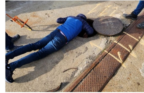
Raman Singh inspects electrical wiring at the foot of Wharf 3.
