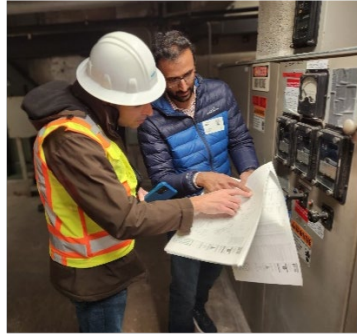
Kamran Kermani (L, M&N) and Raman Singh (R, POSF) examine electrical infrastructure drawings for Pier 68.
