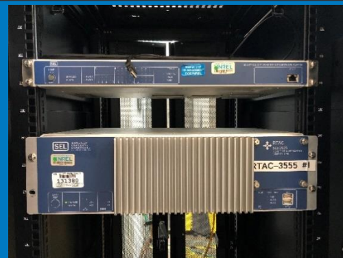
(b) Microgrid controller
