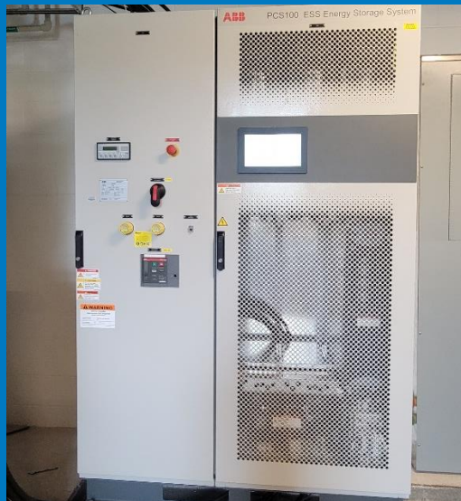
(a) Fuel cell inverter
