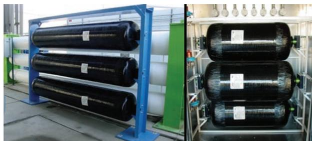
**FIGURE 4.** Three-Bank Hydrogen Cascade Using Composite Pressure Vessels
